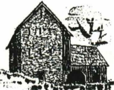
BANK BARN Example of Pennsylvania German construction. Built into a bank for animal protection during winter.
