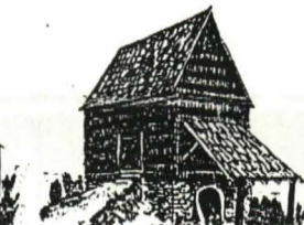
NORTH CAROLINA LOG TOBACCO BARN Unchinked or uncalked log barn with drying oven beneath. Used loft poles to hang tobacco.
