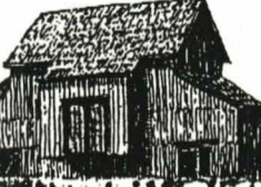
OHIO BARN WITH THRESHING-BAY All wood construction from Ohio's once tall forests. Featured large threshing bay for storing grain.
