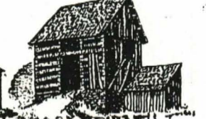
LOG BARN WITH CLAPBOARD SIDING Log barns, inexpensive and efficient, remained popular longer than did log dwellings.
