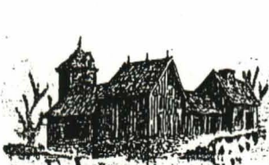
NEW ENGLAND CONNECTING BARN Example of continuous architecture. Farmers could accomplish chores in winter without going outside.
