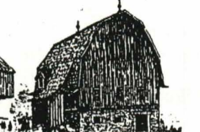
DUTCH GAMBREL ROOF BARN Extension of roof called a "Dutch Knuckle." Barn door above opened onto threshing floor below.
