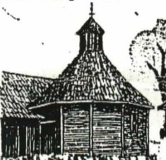
NEW YORK CLAPBOARD BARN Built in the utopian shape of the perfect circle.
