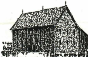
FIELDSTONE BARN Features vertical slits for ventilation. Built from fieldstone. Indicates Dutch-German influence.
